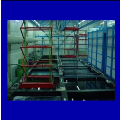
Surface Treatment Plant
